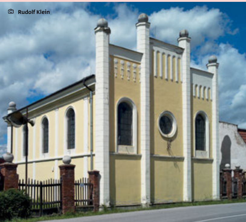
▲ The synagogue was built in 1875 and repaired after a fire in 1905-1906. Its interior still contains a Torah ark, a women's gallery on cast iron columns, and the original rich Moorish ceiling painting. The building serves cultural purposes.
